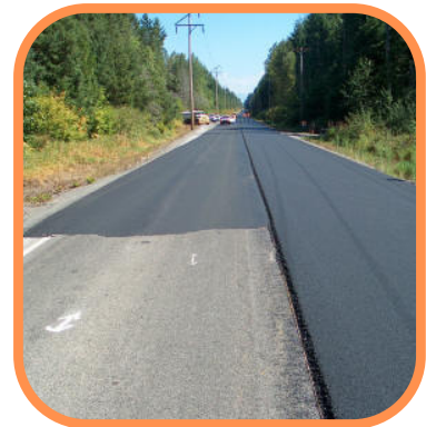
Widen and Overlay
