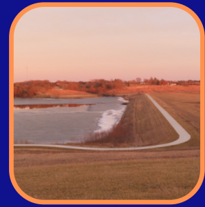
Trail Extension at Little River
