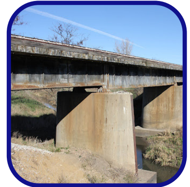
Abandoned Railroad Bridge Replacement in Adair County
