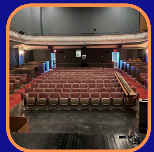
Creston Theater Renovations
