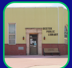
Facade Renovations at the Dexter Library
