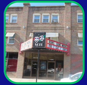
SCIT Theater Renovations
