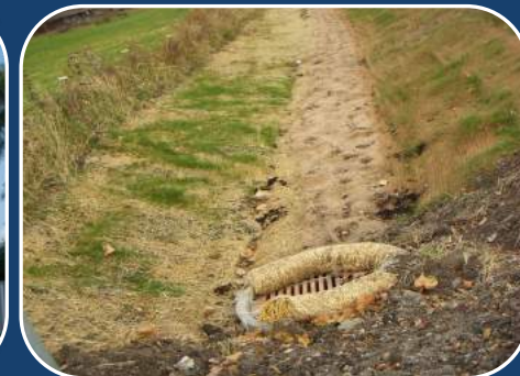
Murray storm water improvements
